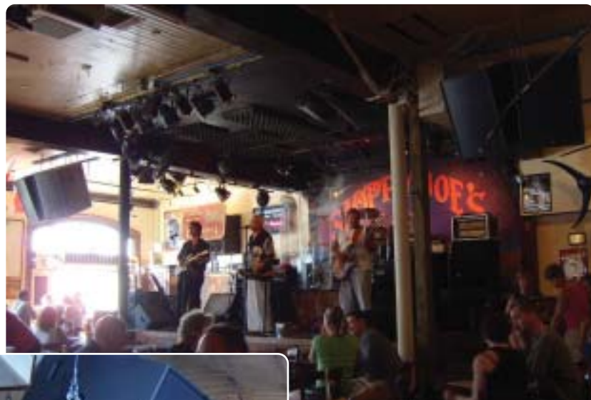
In Sloppy Joe's main room, there are two Martin Audio W8C compact, 3-way, mid-high cabinets per side of the stage flown with a Blackline S218 dual-driver vented sub-bass cabinet under the stage on each side.
