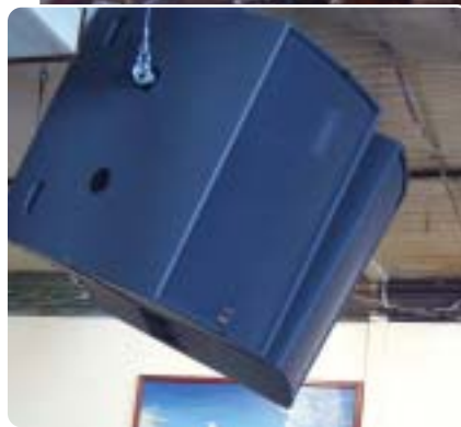
In Sloppy Joe's main room, there are two Martin Audio W8C compact, 3-way, mid-high cabinets per side of the stage flown with a Blackline S218 dual-driver vented sub-bass cabinet under the stage on each side.
